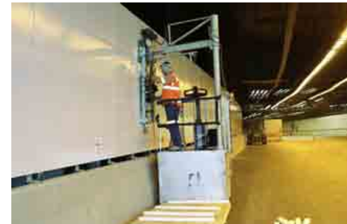
Tunnel installation of flat panels
