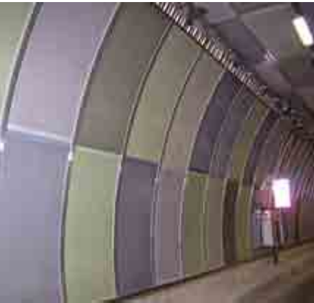
Soundproofing panels | Tunnel Dogana Como | Italy
