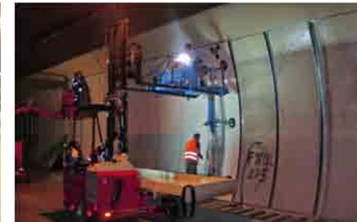
Tunnel installation of curved panels
