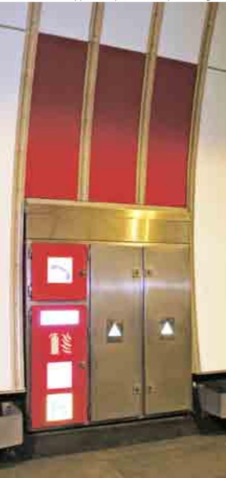
Safety panel box | Cuilfail Tunnel | United Kingdom
