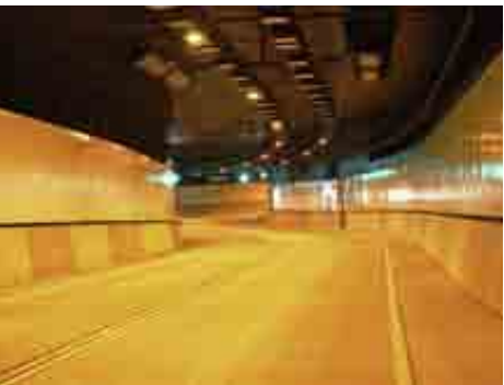
Tunnel Northern Busway - Airport Link | Brisbane | Australien
