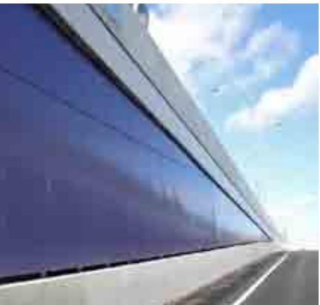
Tunnel Northern Busway - Airport Link | Brisbane | Australien
