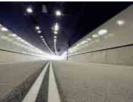
Tunnel Northern Busway - Airport Link | Brisbane | Australien
