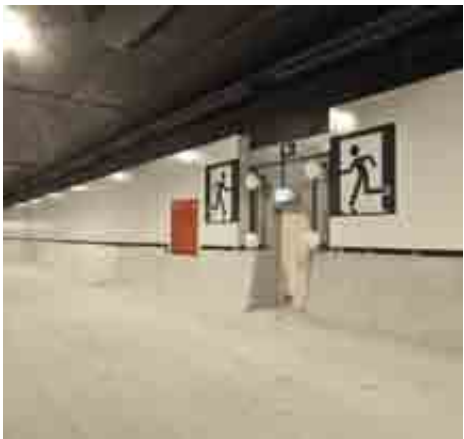
Tunnel Northern Busway - Airport Link | Brisbane | Australien
