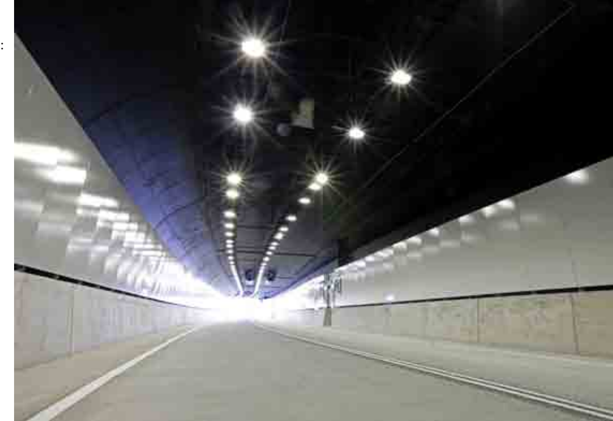
Tunnel Northern Busway - Airport Link | Brisbane | Australien
